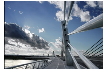
Drava Bridge, Ptuj, SLO
