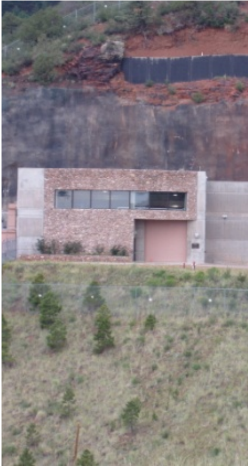
Stanley Canyon Water Purification Facility
