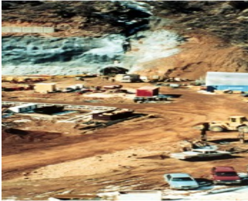
View of tunnel portal at Stanley Canyon
