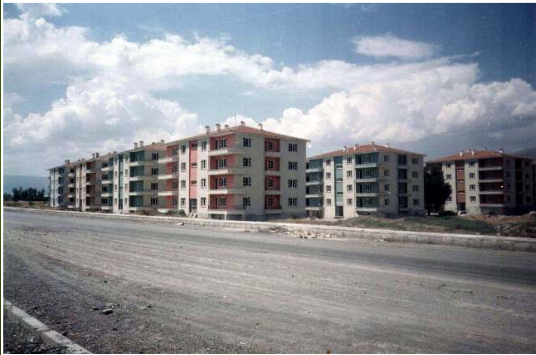
A view from completed Cooperative Apartments
