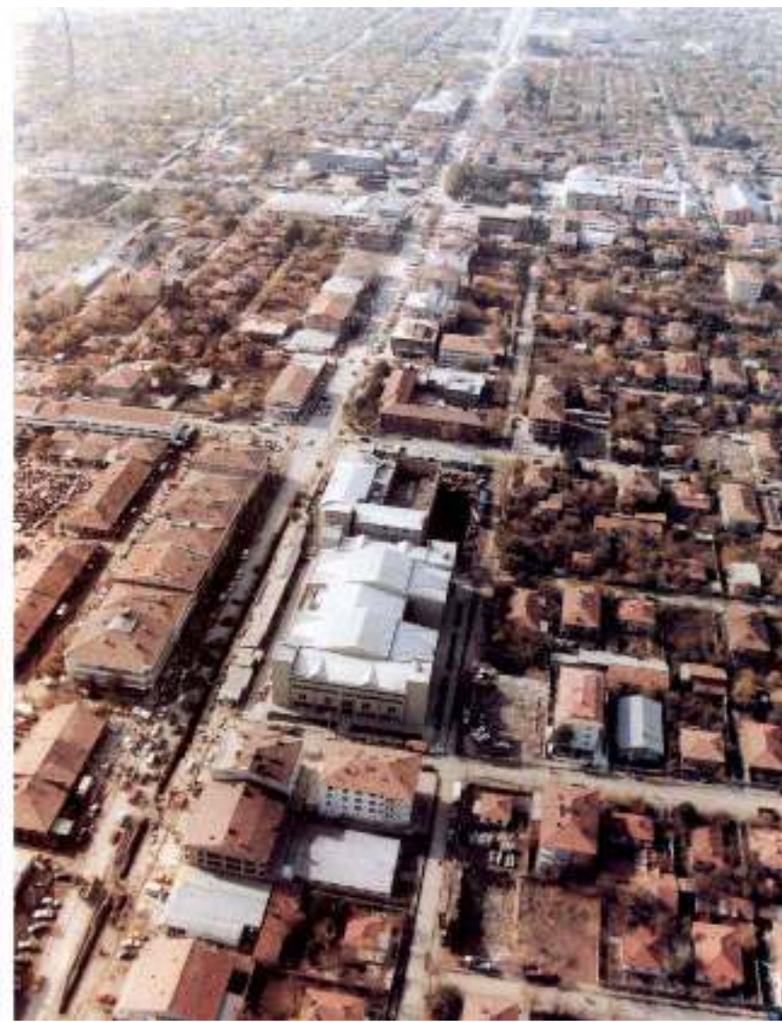
A view of Erzincan in 1995 after rehabilitation and reconstruction
