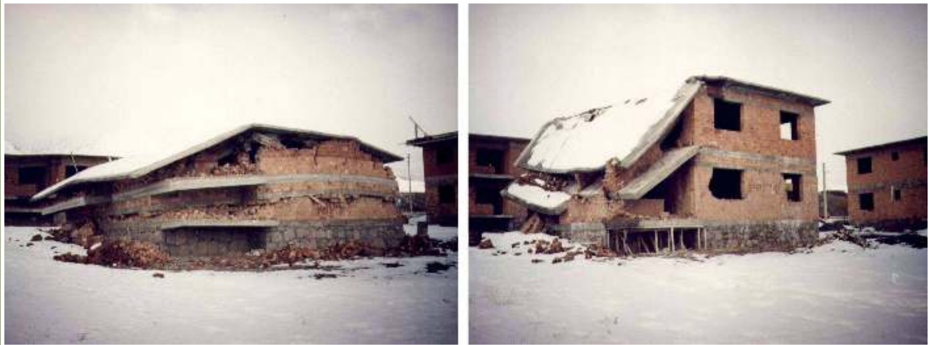
Masonry Houses collapsed due to Earthquake
