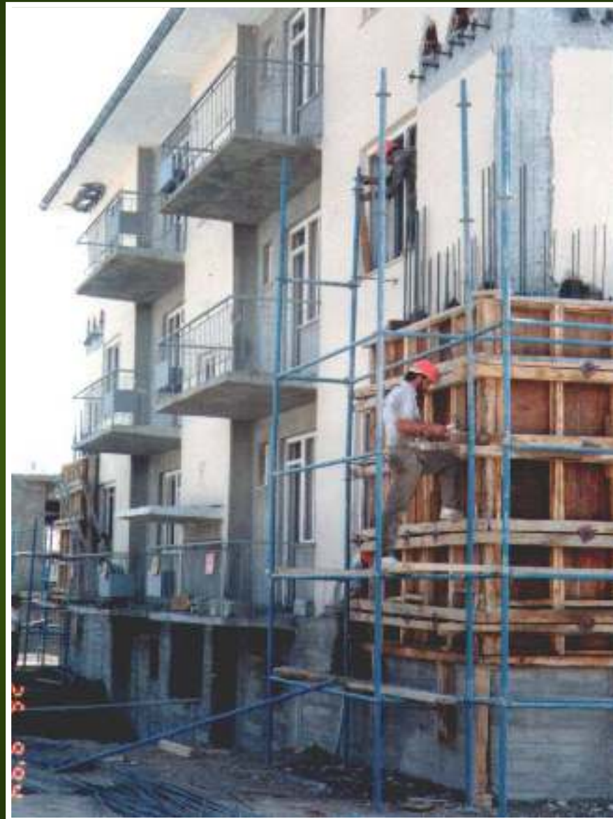
A view from shear wall construction
