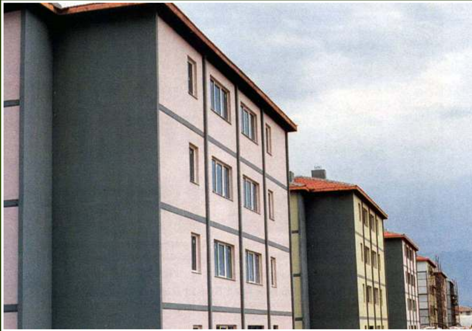
Emergency Repair, Rehabilitation and Reconstruction by the Ministry of Public Works and Settlement
