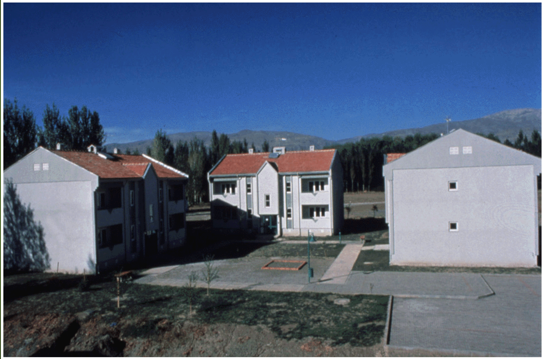
A courtyard protected from the wind and oriented to sunlight
