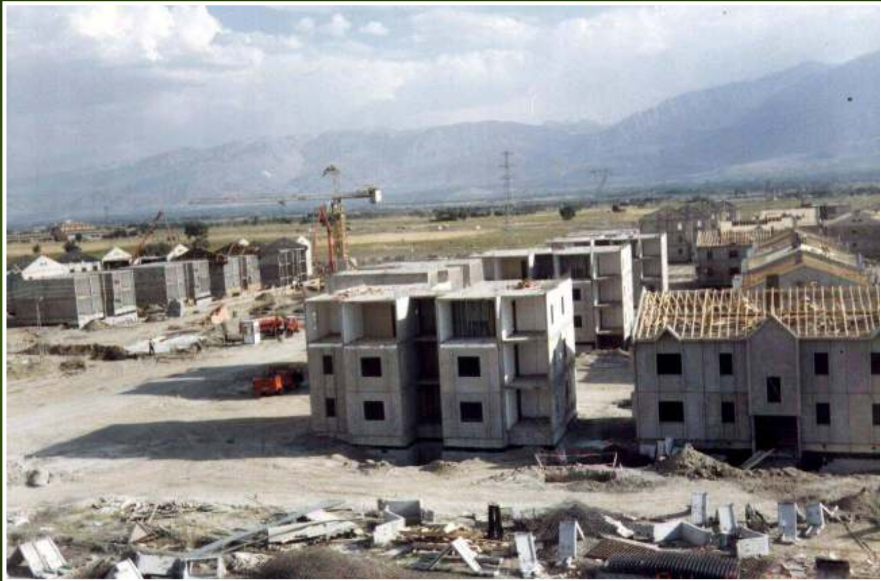
Rapid Construction System – Tunnel Shuttering
